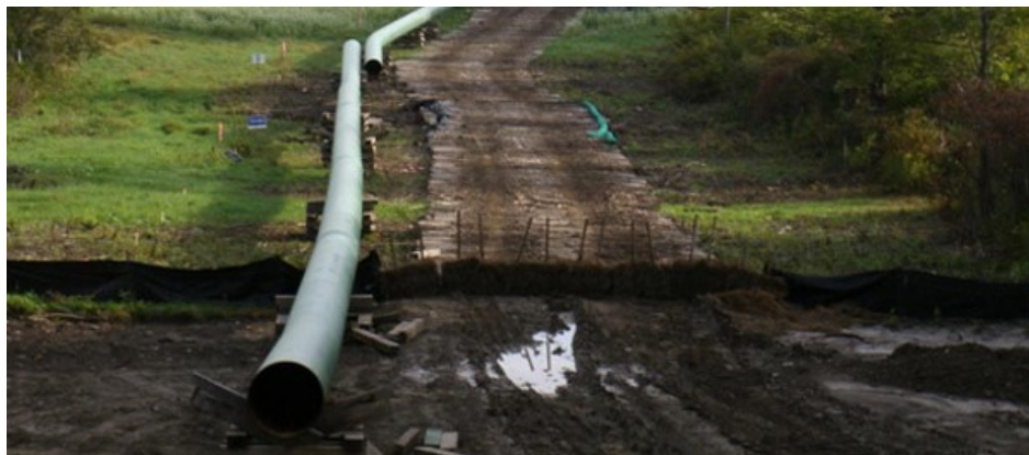
Empire Pipeline Tioga County Extension | National Fuel Gas
