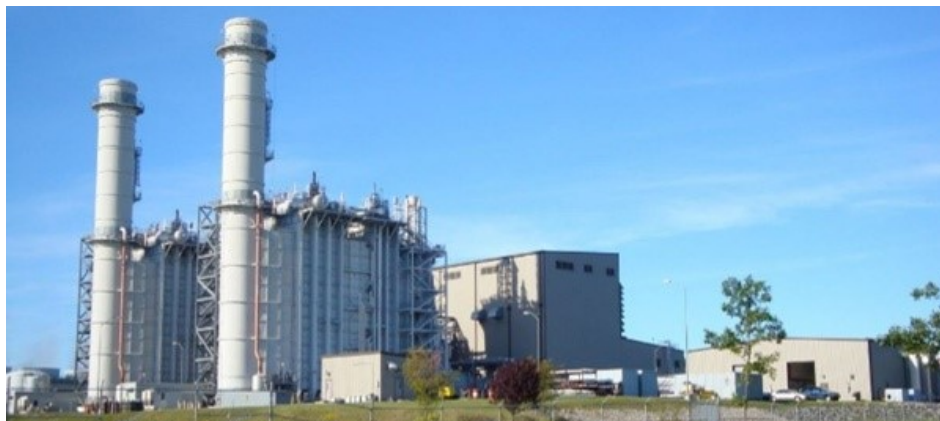
Rhode Island State Energy Center | Entergy
